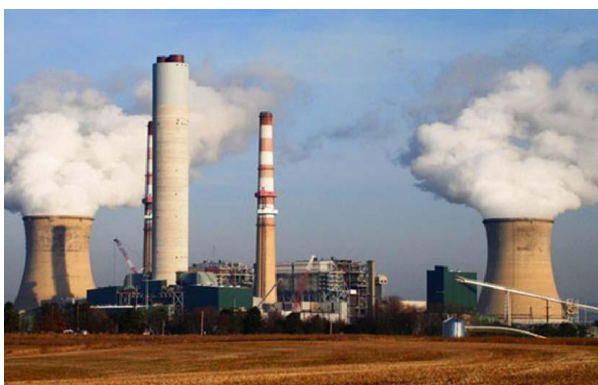
Fig. 1.1: Cantilever Steel Chimney
